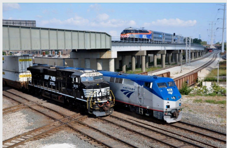
A new rail flyover at 63rd and State in Chicago that eliminated an at-grade crossing as part of the CREATE project, bringing benefits to urban and rural communities alike across the region, state, and country. Photo by Mark Llanuza.
