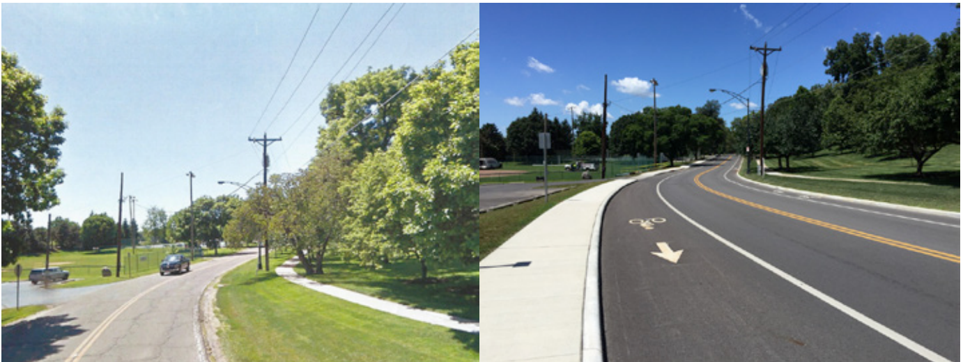
Goodale Boulevard, in Grandview Heights, lacking safe access for those traveling on foot, bicycle, and wheelchair in the before photo at left. Goodale Boulevard, right, after the addition of sidewalks and bicycle lanes.
