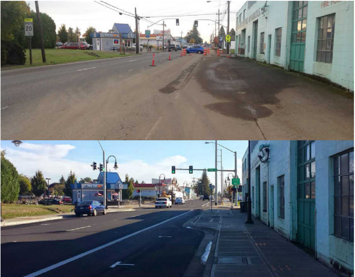
The RFF program funded new wide sidewalks, lighting, and safer crossings for people traveling on foot, as well as bicycle lanes, on Baseline St. in Cornelius, OR. Photos courtesy of Metro.
