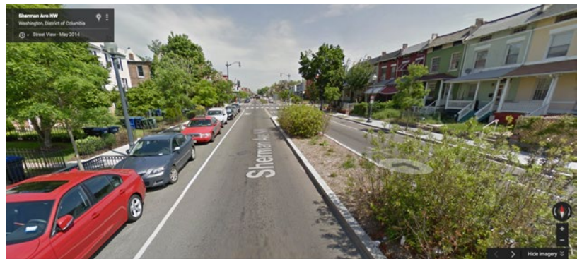
With wide lanes and excess capacity, Sherman Ave. in Washington, DC was unsafe for everyone who used it and was retrofitted to add a median, crosswalks, and bulbouts to improve safety and functionality for all. Imagery via Google Maps.
