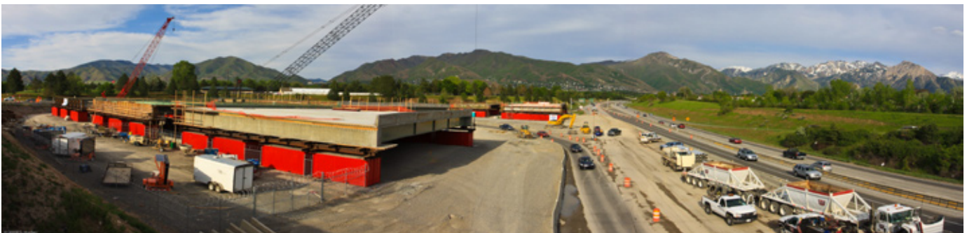
UDOT "bridge farming" on I-15. 70 percent of new gas tax revenues will be controlled by the state and dedicated to road projects. Flickr photo courtesy of Shaan Hurley https://www.flickr.com/photos/btl/2700839269
