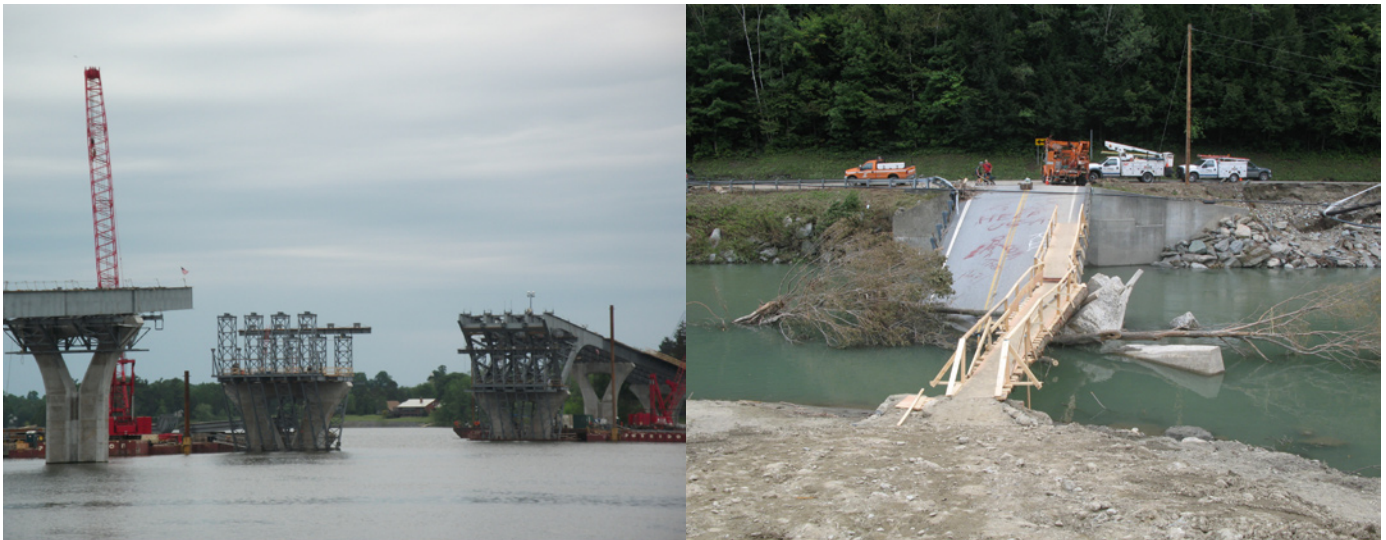
The Crown Point Bridge during replacement in 2011 (left) and the Route 73/Route 100 bridge in Rochester, Vermont after its collapse during Tropical Storm Irene in August 2011. Left Flickr photo by Doug Kerr. https://www.flickr.com/photos/dougkerr/6785141518 Right Flickr photo by belvidesigns. https://www.flickr.com/photos/45631932@N03/6106160352
