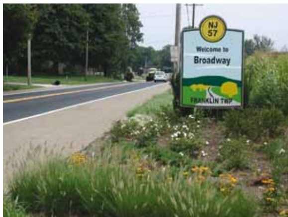
After the corridor project, the streets feature wide shoulders and attractive landscaping.
